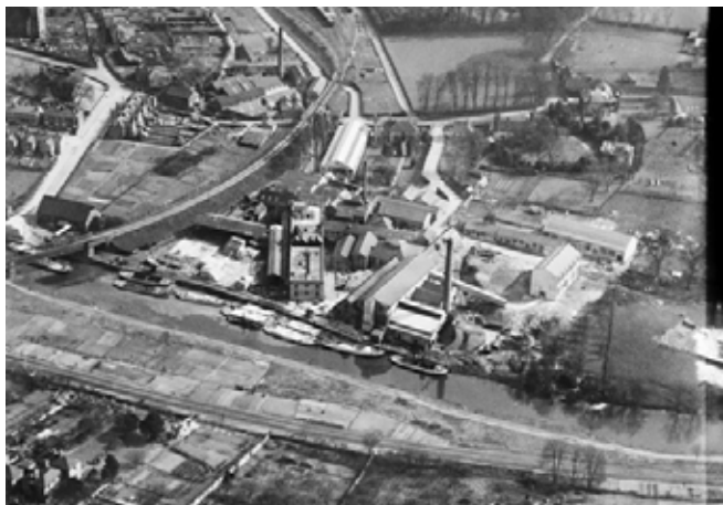
Figure 4.4: Bridge Mill Viewed from the South
