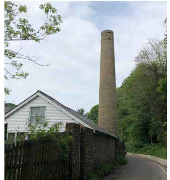
Figure 11.11: The great brick chimney at Hayle Mill
