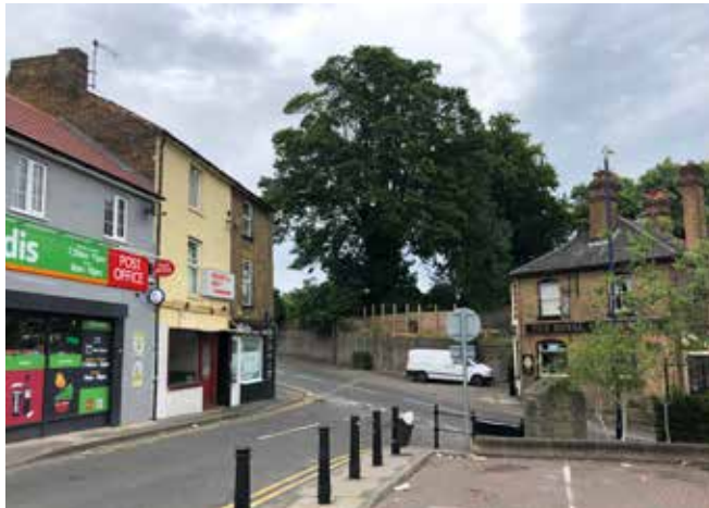
Figure 2.6: Contemporary view of Church Street, most of the historic buildings have been lost, however, the street retains its original layout.
