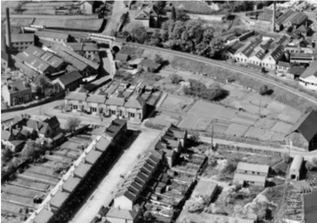
Figure 3.4: Aerial view of the Junction of Beaconfield and Wharf Roads
