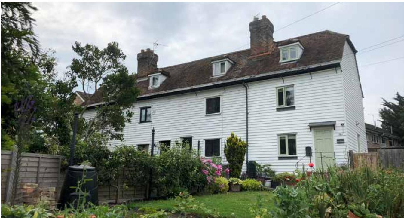
Figure 4.8: Early 19th Century, Grade II Listed Agricultural Workers' Cottages
