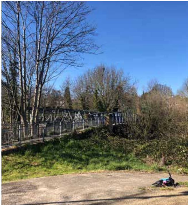
Figure 3.12: View of footbridge over the River Medway
