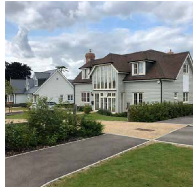
Figure 8.4: Timber cladding and traditional clay tiles borrow from local agricultural and paper mill worker cottages.
