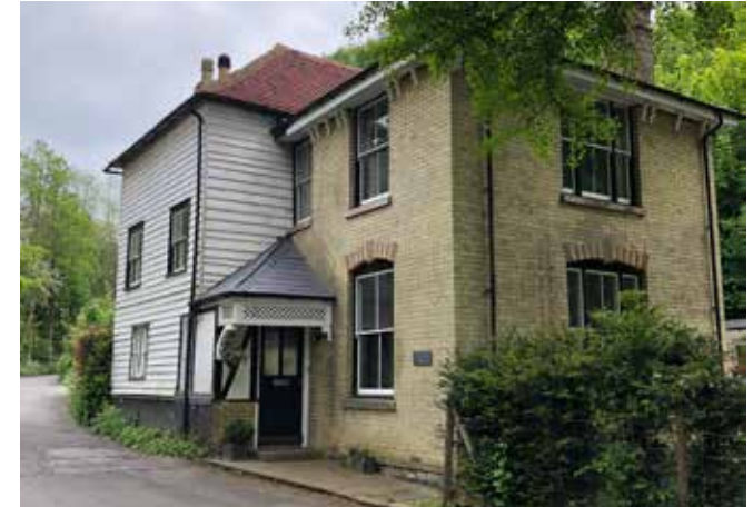
Figure 11.3: Crisbrook House, with drying building in timber.
