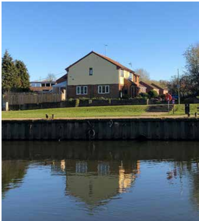
Figure 4.2: View of the Loose Stream Outlet, hardly visible in the bank wall.
