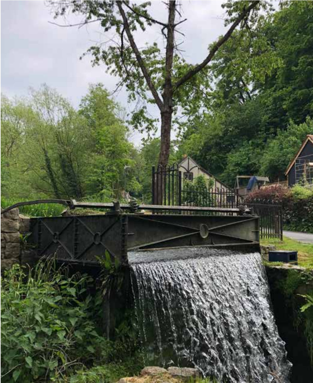
Figure 9.8: Remains of Lower Crisbrook Mill
