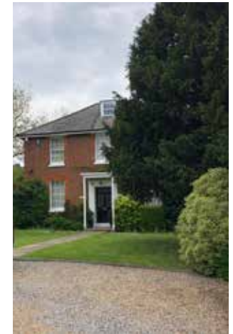
Figure 2.10: Grassmere House, Grade II Listed.
