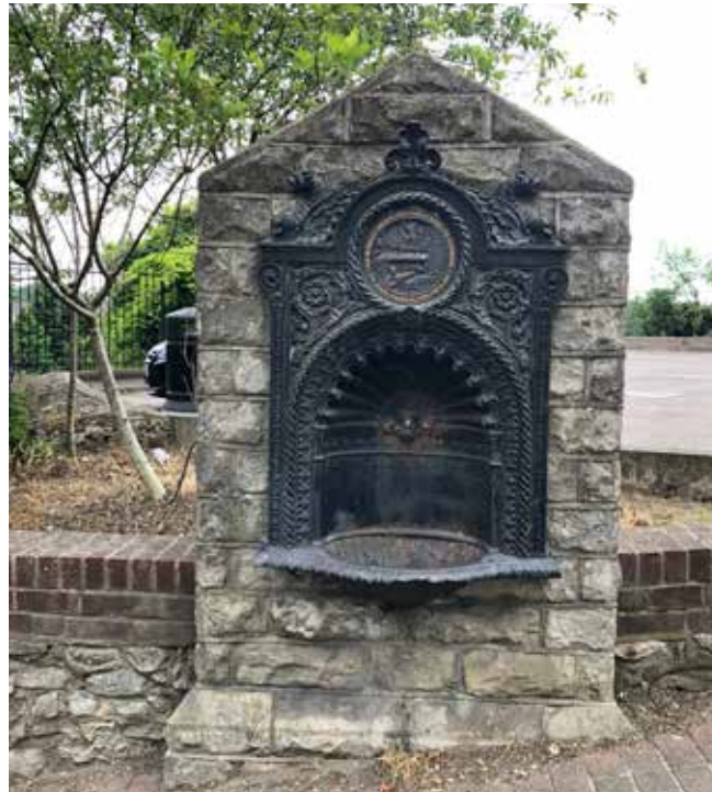
Figure 11.10: Drinking Fountain, corner of Church Street and Tovil Hill
