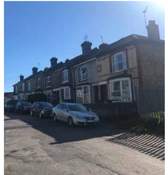
Figure 3.9: Wharf Road houses built for Paper Mill Workers in 1905.
