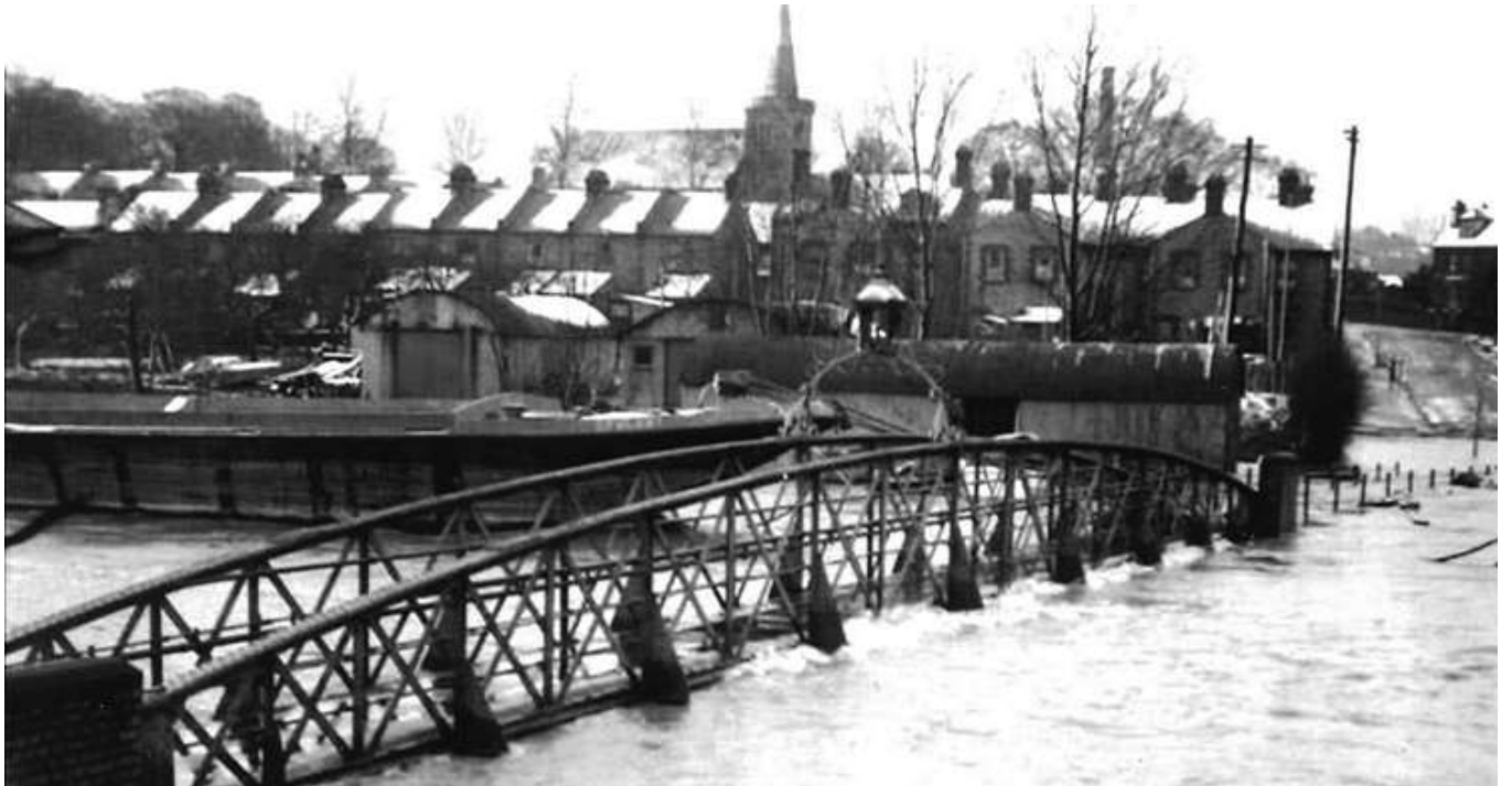
Figure 3.13: View of the footbridge during a flood, with the rear of Beaconsfield Road Houses and St. Stephen's Church in the distance
