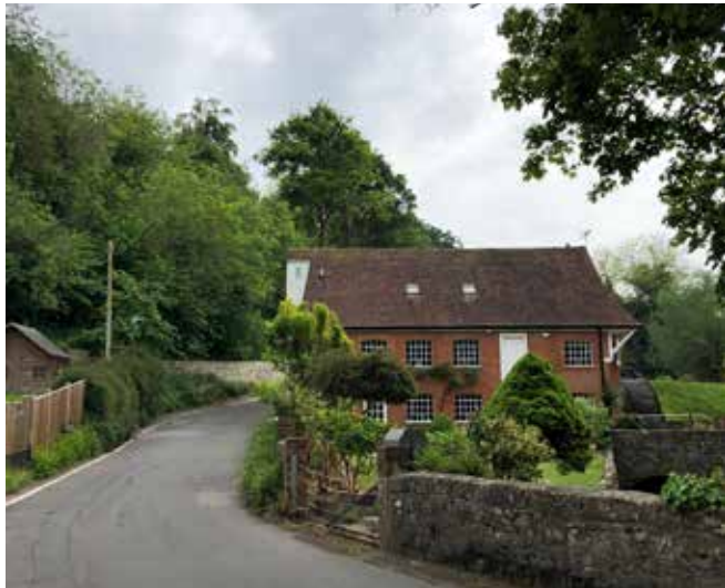
Figure 9.4: Upper Crisbrook Mill, which retains its waterwheel
