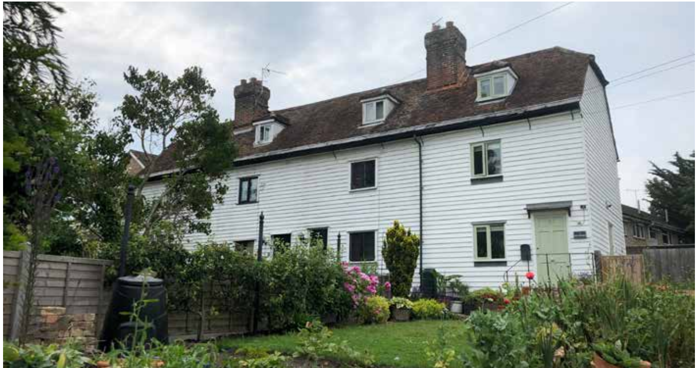
Figure 11.5: Workers' Cottages, Tovil Green Lane
