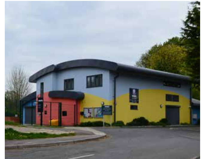
Figure 5.6: Tovil Community Centre of questionable architectural merit
