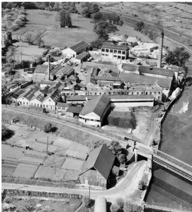
Figure 4.7: Detail of Bridge Mill
