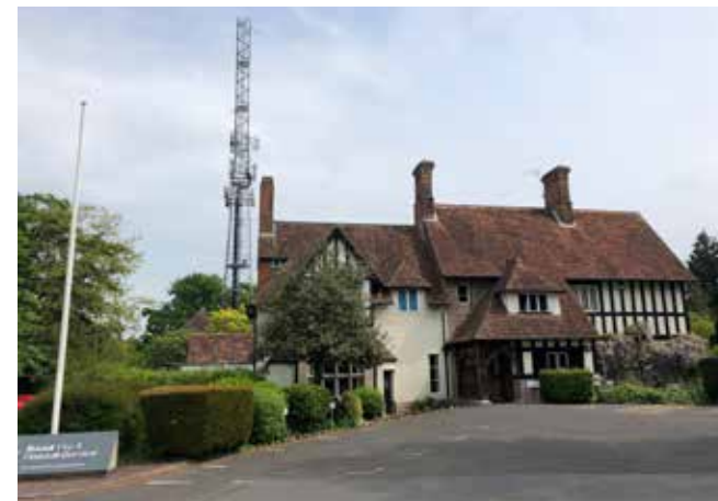
Figure 10.5: Kent Fire & Rescue HQ concealing the bulk of the complex
