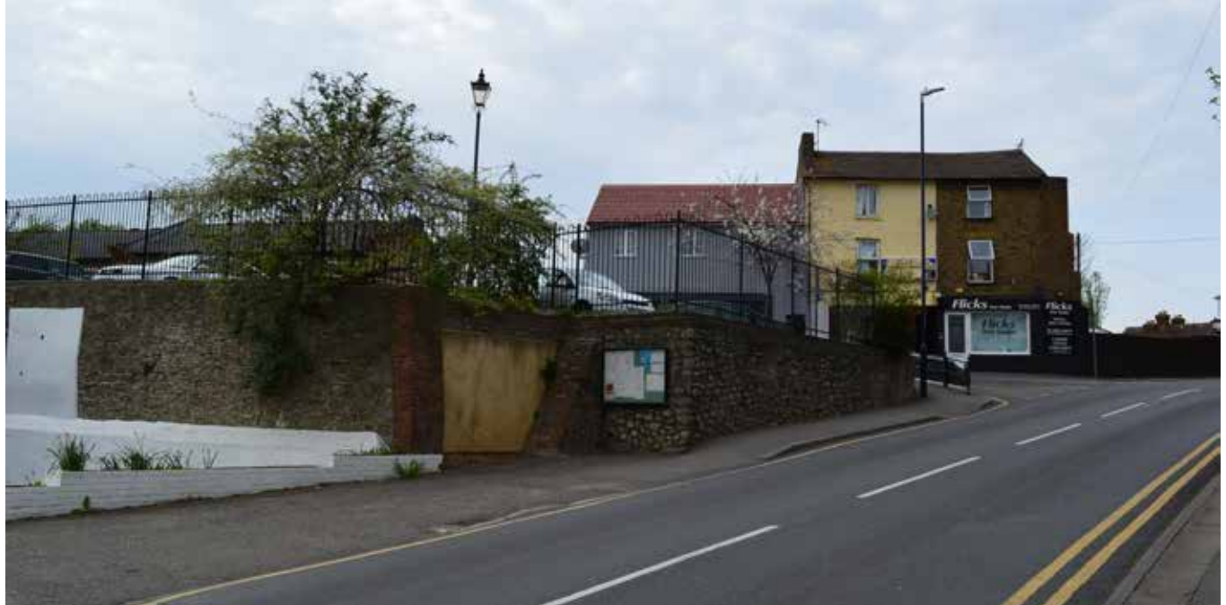
Figure 2.7: View of the junction of Church Street and Tovil Hill, where some of the original historic structures remain
