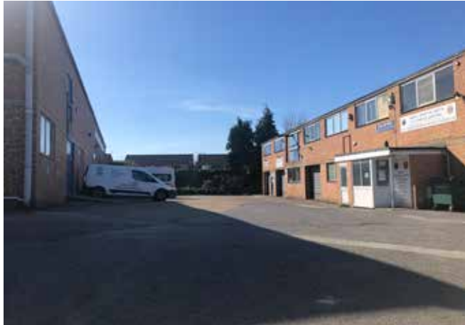
Figure 3.9: View of Wharf Road Industrial Units
